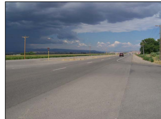
Hwy. 92 looking east
